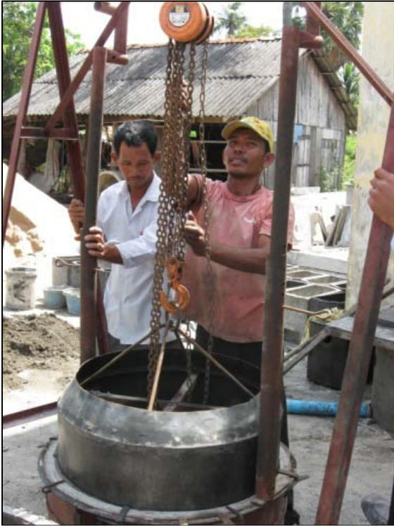
Removing the inner mould during concrete ring construction
