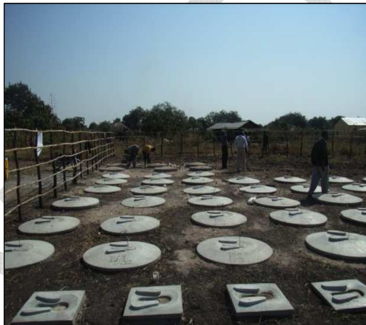
Demonstration Center, Maravia District, Tete Province, Mozambique
